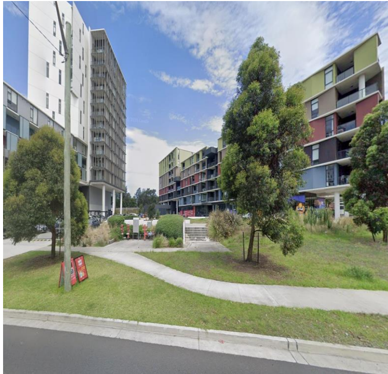
Figure 1: 1-5 Link Road and 132-136 Epsom Road, Zetland, viewed from the west
